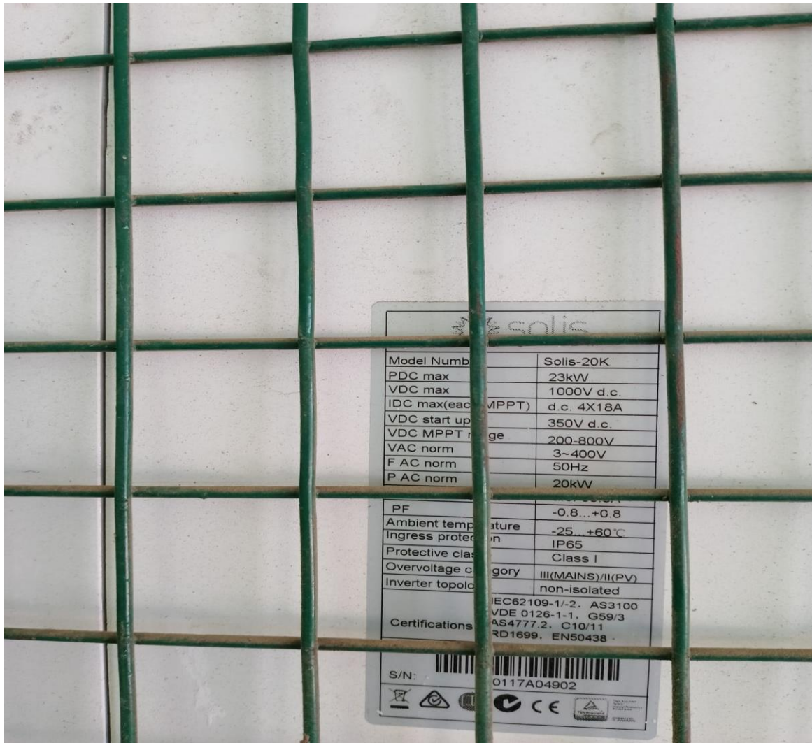
Details of the Solar Power Unit
