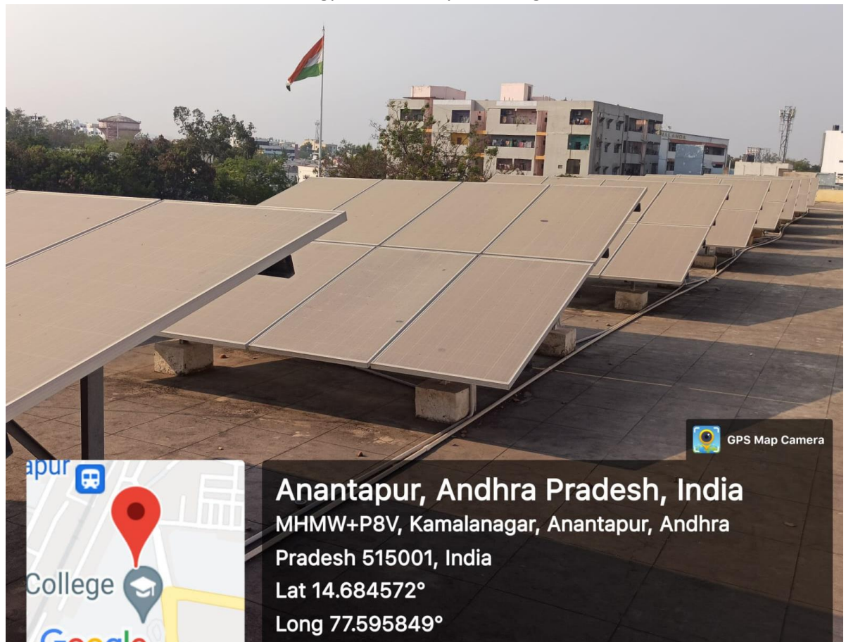
Solar Pannels on the Commerce Block
