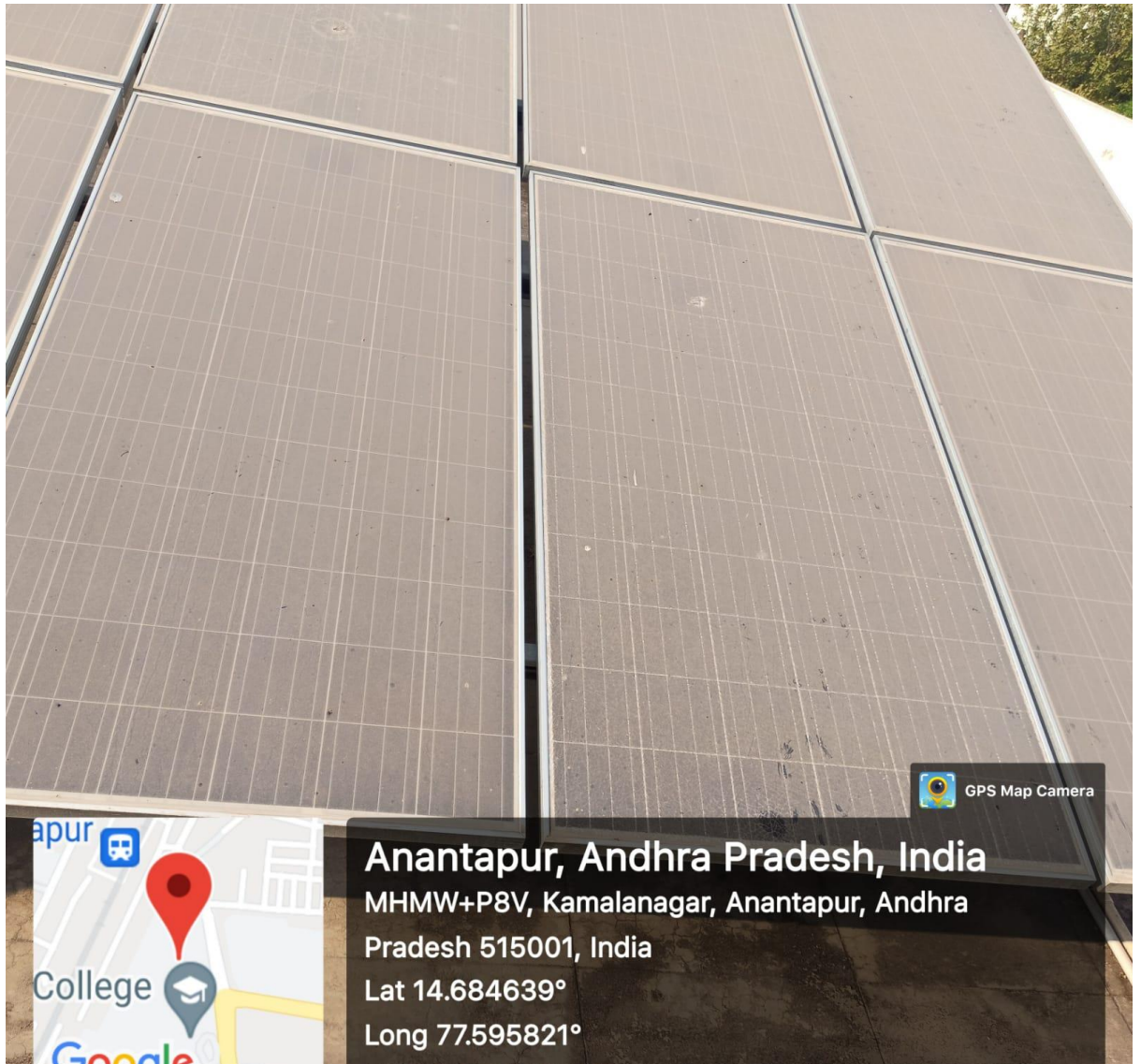
Solar panels on the commerce block
